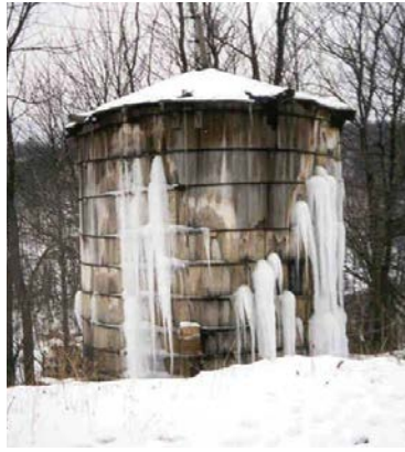
Elkhorn water tower was built in the 1950s.
