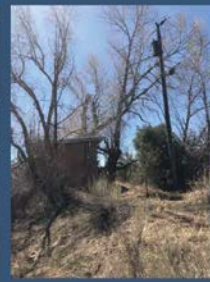
Well 1 Well House
