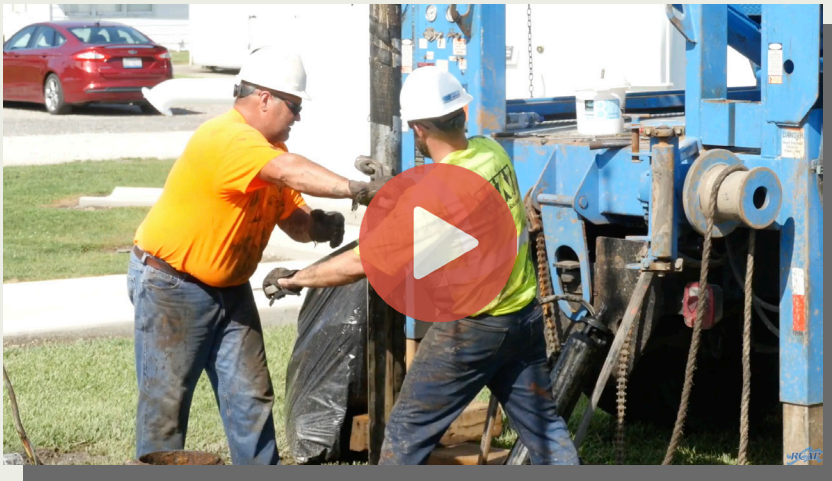
Potholing for Lead Service Line Verification
